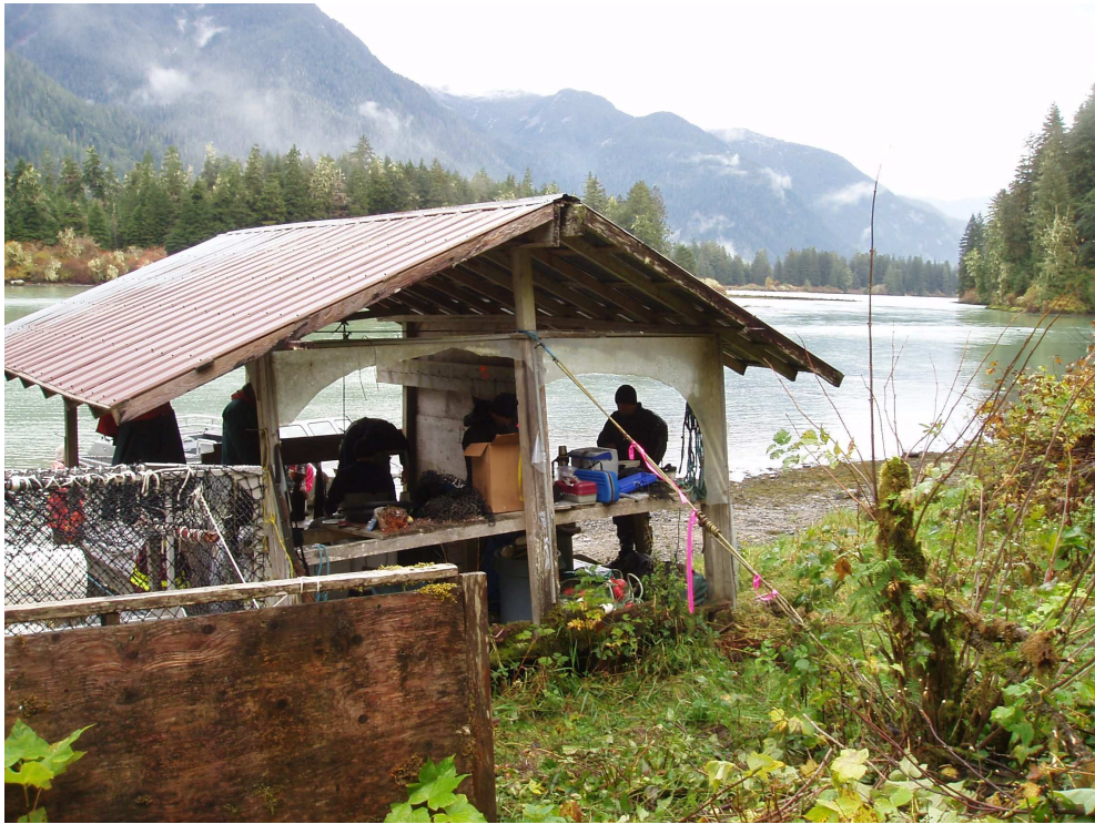
Eggtake shed with guy wire to secure it until repairs can be done
